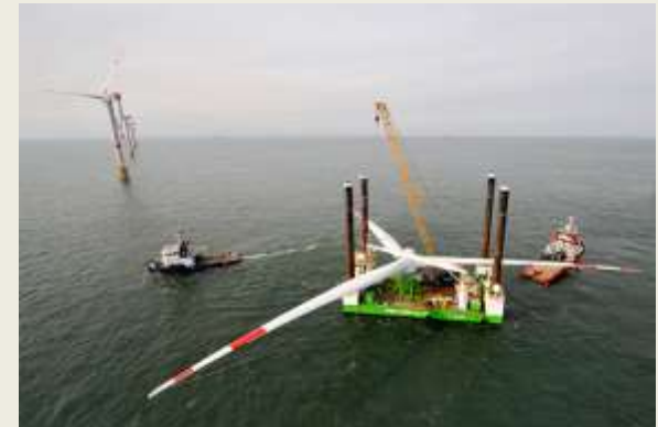
©2008 by Jan Oelker/REpower Systems
